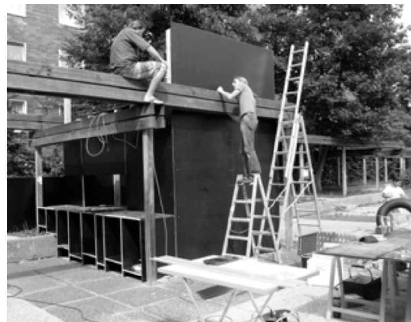
Figure 23.3 Temporary pavilion in progress, Hustadt Project, Actions, 2008–2011, Bochum, Germany
