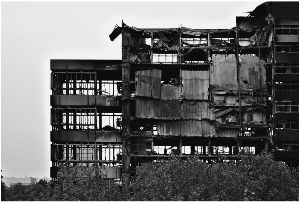
5. TU-Delft Faculty of Architecture After Fire, May 2008. (Photo by Sjors van Berkel courtesy of TU Delft.)
